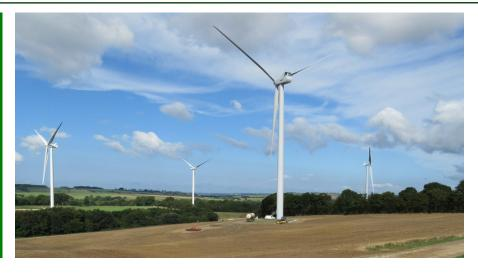
Design and Construct contract for Civil and Ancillary Works for a 9 turbine wind farm site constructed in largely undulating pastoral farmland near Crediton in Devon. The wind turbines procured for the site by RES were Vestas V90 2.0 MW units with 120m tip height. Turbine erection was completed in October 2016 and the site was generating electricity by the end of 2016. the installed capacity equates to 18 MW of renewable electricity sufficient to met the needs of 9,000 homes.
